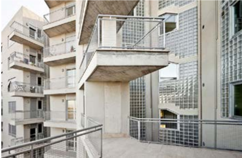
Edeficio 111 , Social Housing, Barcelona, Spain, Photographs by Duccio Malagamba and Adria Goula.
