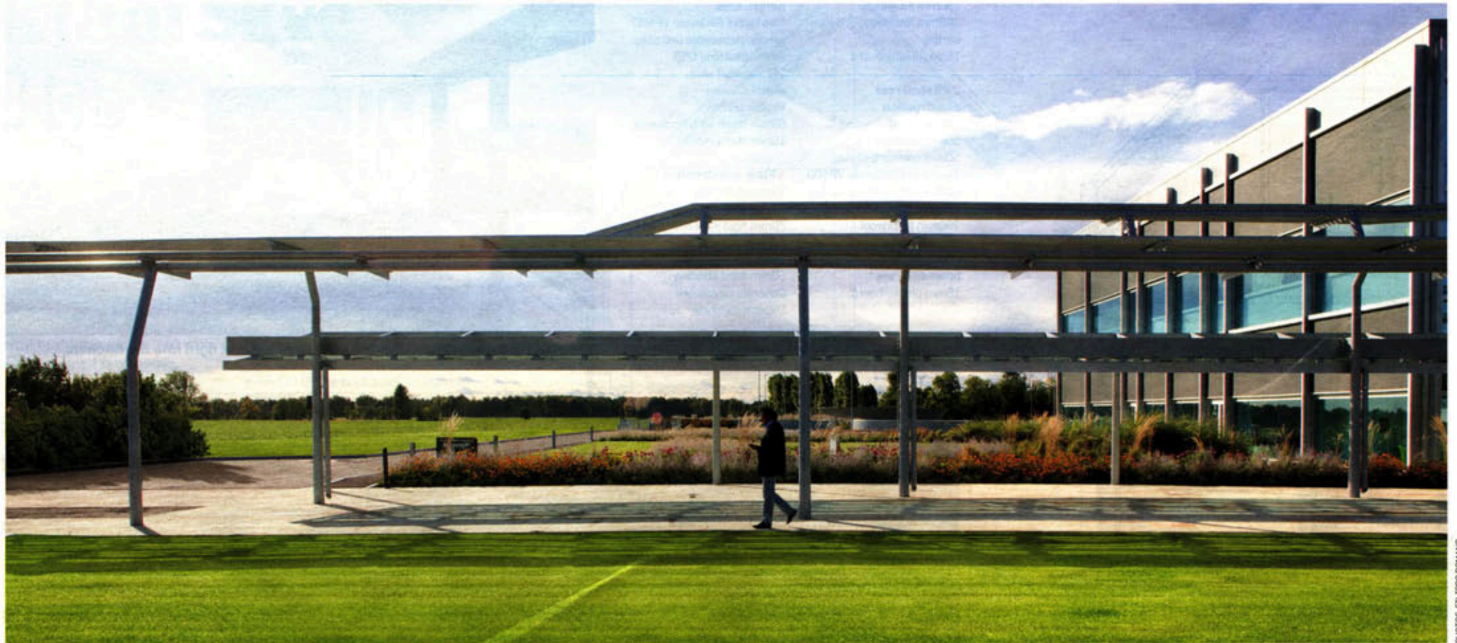
The steel and glass rain pergola extends from the building's facade at a lower level than the shade pergolas to provide a canopy that gives shelter from the weather.
